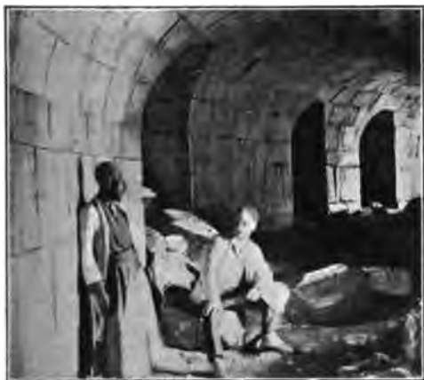
GADARA: VAULTS UNDER SEATS OF THEATRE
